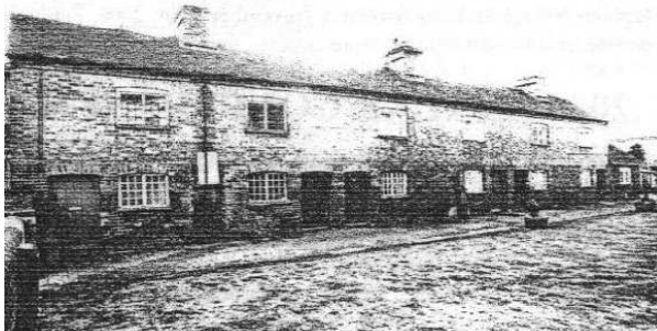
Feoffee Cottages as they were between 1866 and 1976. Note the water pump in the centre.
